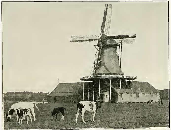
FIG. 263. — A windmill in The Netherlands, used for pumping out the water from the land inclosed in dikes.
